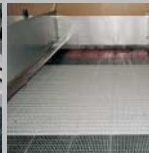
4. Heat pads, floor panels and slat sections are fitted.
