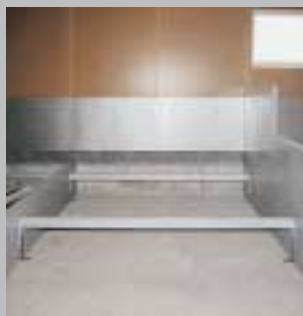
2. Cross beams are installed at floor level, either suspended between partitions or resting on the channel floor.
