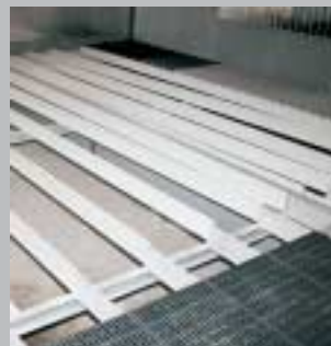
3. Floor supports are mounted on the cross beams.
