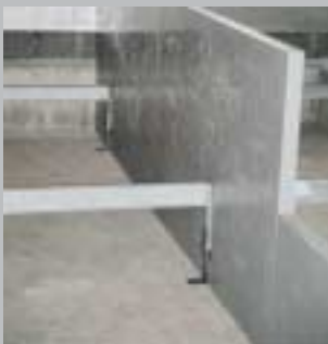
1. Multiflex cellular panels are mounted on the channel floor using fittings.
